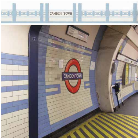
Fig. 6. Above: Section of the original tile scheme at Camden Town (Rose 2007, pull out “The Hampstead Stations”). Below: Retiled platform at Camden Town (author’s photo).
