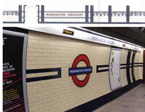
Fig. 4. Above: Section of the original tile scheme at Mornington Crescent (Rose 2007, pull out "The Hampstead Stations"). Below: Retiled platform at Mornington Crescent (author's photo).
