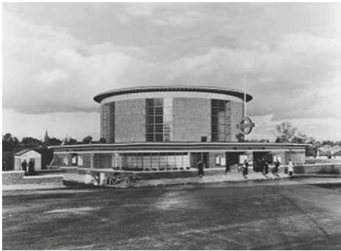
Fig. 1: Examples of London Underground stations designed by architect Charles Holden. From top: Chiswick Park (photographed by Topical Press 12 Oct 1932, LTM U11500); Turnpike Lane (photographed by Topical Press Jan 1933 - Mar 1933, LTM U11887); Arnos Grove (unknown photographer 1932, LTM unknown image number).
