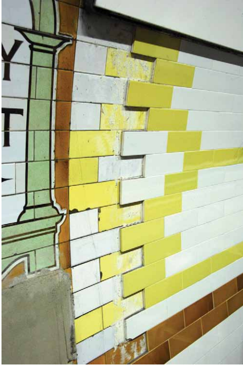
Fig. 5. Over-tiling at Covent Garden (photo courtesy of Douglas Rose, 2008: http://www.dougrose.co.uk/index_tiles.htm [accessed October 2012]).
