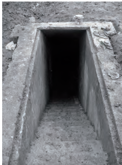
Figure 2. The entrance of the shelter, following excavation.
