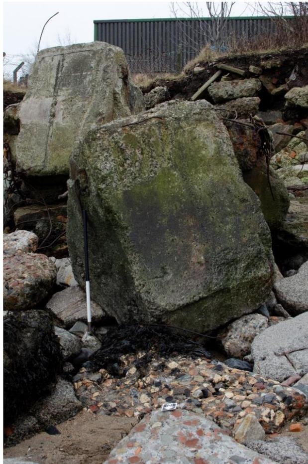
**Figure 5:** Large triangular 1950s/60s concrete foundations lying on their sides (the piece in the foreground has bent steel rebar at right, indicating the original top surface). Located on the eastern bay of Royston Beach. The reclaimed land and a disused warehouse lies behind. One metre scale. Photograph by the author. CC BY-SA-NC 4.0.
