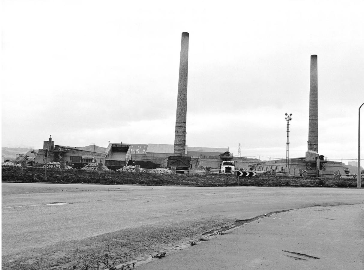
**Figure 15:** Niddrie Brickworks in October 1974. View from northeast showing Hoffman brick kilns and chimneys. This area is now home to Fort Kinnaird shopping centre. Image: 000-000-186-212-R ©Crown Copyright: HES.
