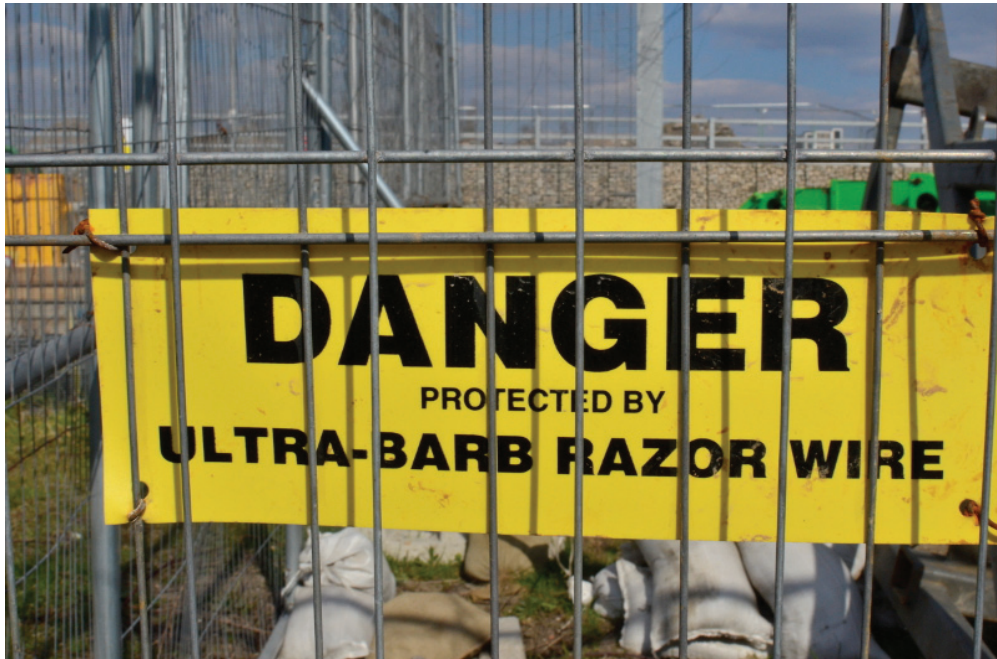
Figure 14: ‘Ultra-Barb’ warning sign on the temporary fencing. Photograph: J. Gardner.
