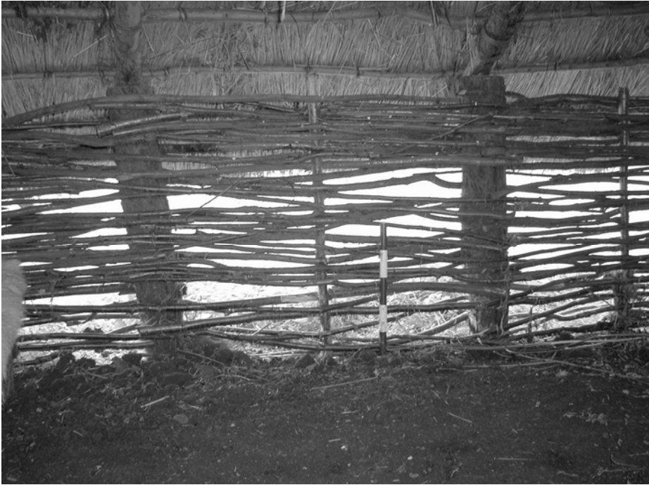
Figure 3. The familiar wattle wall. Materials and technologies clearly discernable and easily ‘readable’. ‘Iron Age Roundhouse’ Flag Fen, Cambridgeshire.
