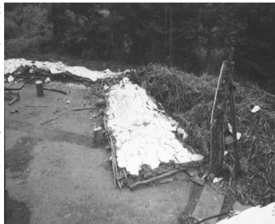
Figure 7. Obtrusiveness: total collapse; the wall of this roundhouse, which stood near Cardiff, Wales, can no longer be encountered in the role for which it was intended. [ http://www.theroundhouse.org/a/RH1/1decon/ga129lg.jpg ] [accessed 17.02.2003] Courtesy of Dafydd Wiliam.
