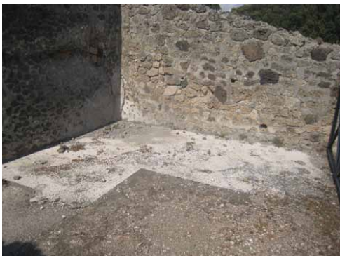
Fig. 8: Not all conservation problems are due to overcrowding. Many of the closed areas suffer from neglect as resources are diverted to the open areas on-site. Mosaic floor in area 13 on Figure 5. Tesserae from mosaic are loose and the surface is rapidly decaying.
